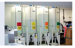
**Note:** Reconstituted acid concentrate should not be stored in the Dry Acid Dissolution tank for longer than two weeks from the date of dissolution.
